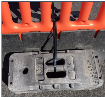
Cable tie Everest Blocks to bracing units as shown.
